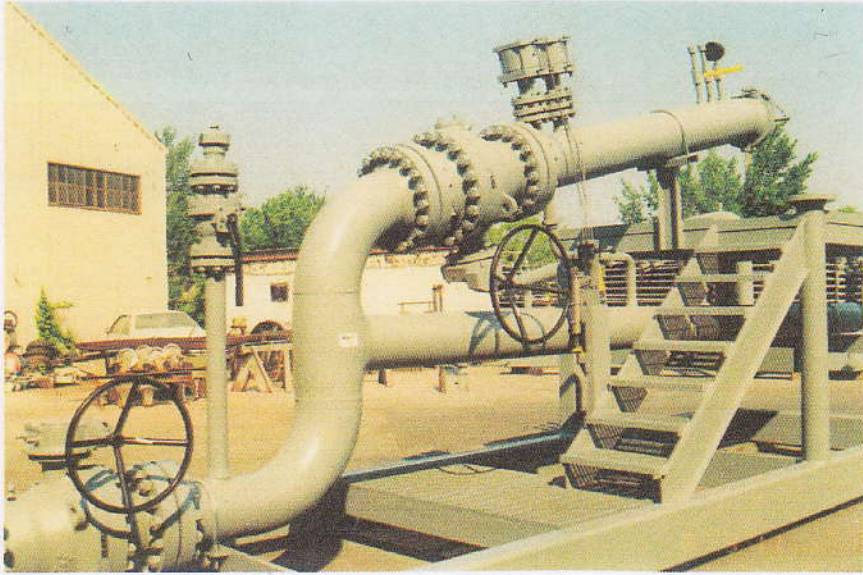
10" Sphere Launcher, skid mounted, with block valve and blow downs.
